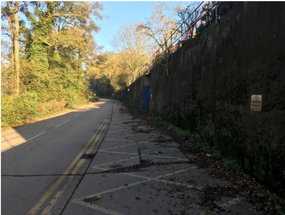
Retaining wall adjacent to Thames Valley Estate Road
